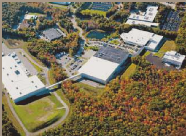
Aerial view of the newly extended Lindt & Sprüngli plant in Stratham, New Hampshire.
