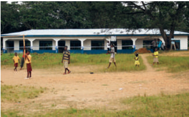
In 2010, a new Junior High School in Dunkwa, Ghana, has opened, which was built with a part of the donations by Lindt & Sprüngli.
